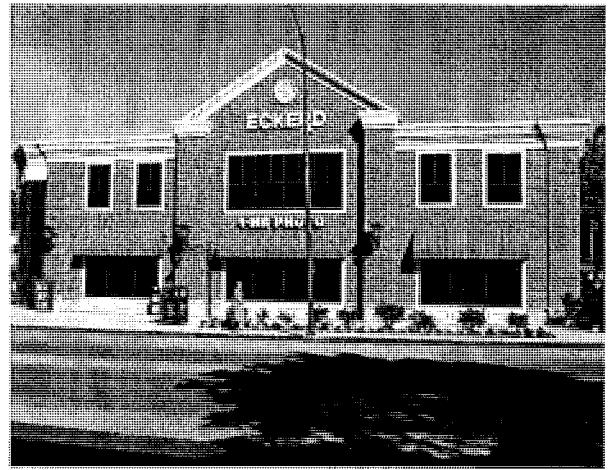
Figure 3.1 Example of building design incorporating successful facade base and roof top treatments. Brick pilasters are used to break massing appropriately. Architectural details such as cornices, awnings, and window casing are used to give the building a "human scale".
