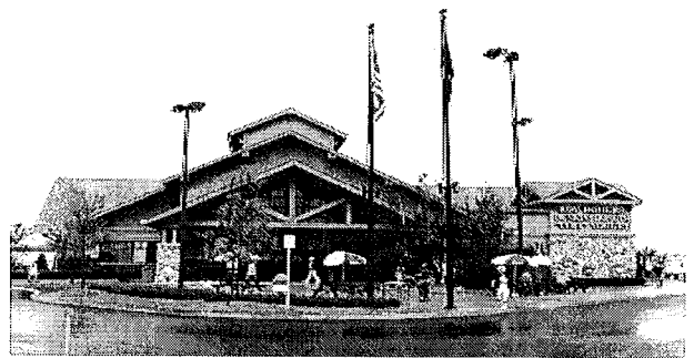
Figure 3.3 Example of design incorporating successful facade base and roof top treatments, and building tenant signage. Design utilizes a variety of roof top treatments and forms to break down the building mass into smaller human scale elements.
