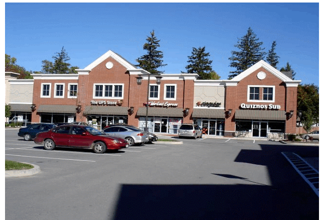
Figure 2.8 Example of In-line Retail design incorporating successful facade base and roof top treatments. A mix of brick and EIFS accent materials, are used to break an otherwise lengthy facade into smaller elements. Architectural details such as cornices, awnings, and window casing are used to give the building a "human scale".
