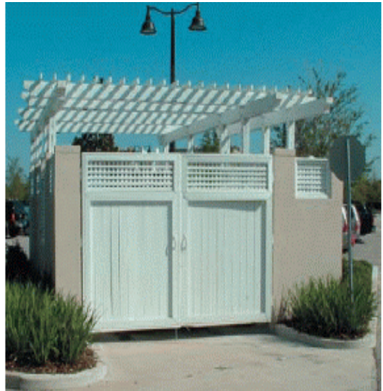
Figure 2.6 Albeit not a fitting architectural style for Grand Island, this is an example of proper dumpster screening and gates utilizing architectural elements to match the style of the main building.
