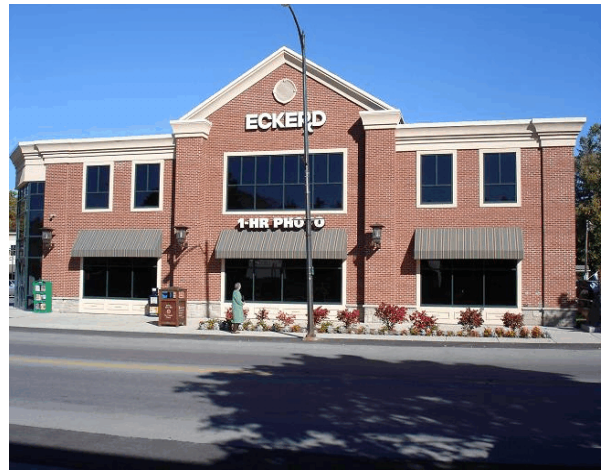
Figure 2.7 Example of building design incorporating successful facade base and roof top treatments. Brick pilasters are used to break massing appropriately. Architectural details such as cornices, awnings, and window casing are used to give the building a “human scale”.
