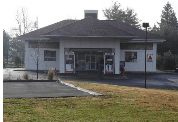
Figure 3.0 Example of Convenience Store and Gas Station with canopy rooflines matching the primary structure without becoming a dominant feature.
